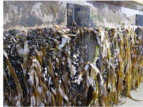
Quagga mussels render water diversion structure inoperable. Imagine what they could do to a pump!
